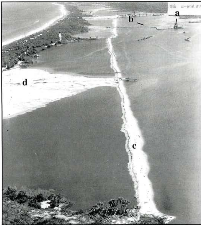
Dredge and dike. Low, oblique aerial view north from Manasota Beach, taken circa 1964-65. Manasota Key Bridge is in the midground. This photo shows dredge (a), pipeline (b), dike or containment wall (c) and back-filled, spoil (d). This phase of dredging the Intracoastal Waterway, with the use of back-filling land along the shoreline, differed from the early dredging where spoil was side-cast in strips or islands parallel to the route taken by the dredge.
