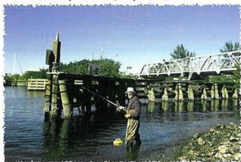
Blackburn Point Bridge
